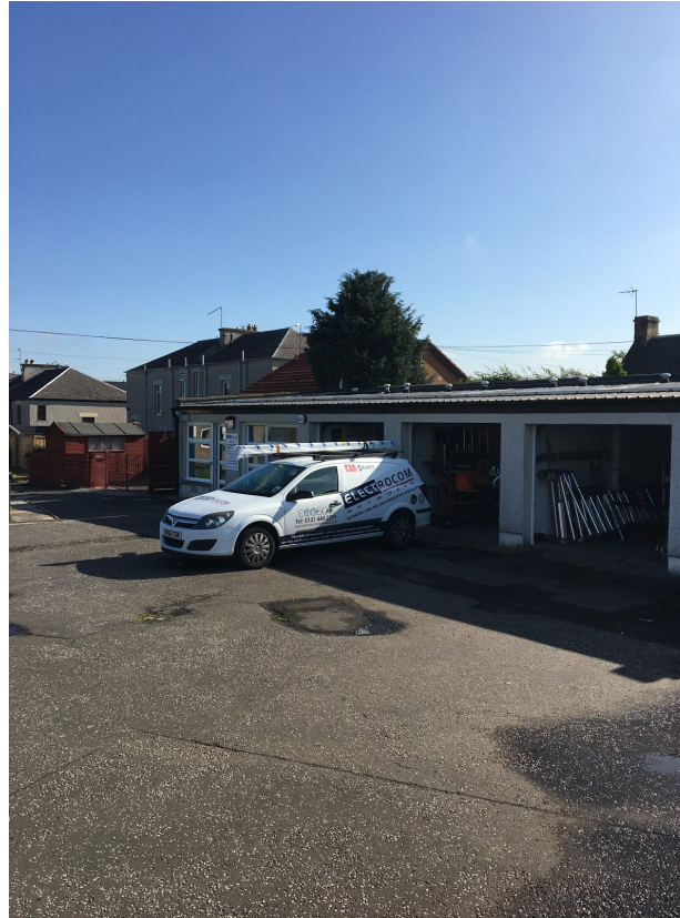
Existing street frontage to property.
